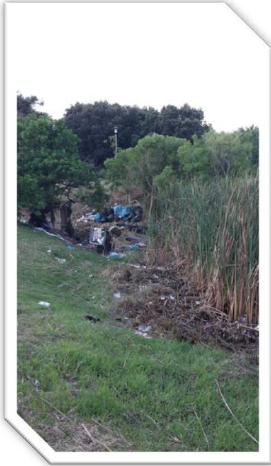
*Unpleasant consequences of a poorly managed sustainable urban drainage project. Removing the reeds reveals the problem of litter, blockages and accumulation of biomass. Photo: Kevin Winter 25 October 2014)*
